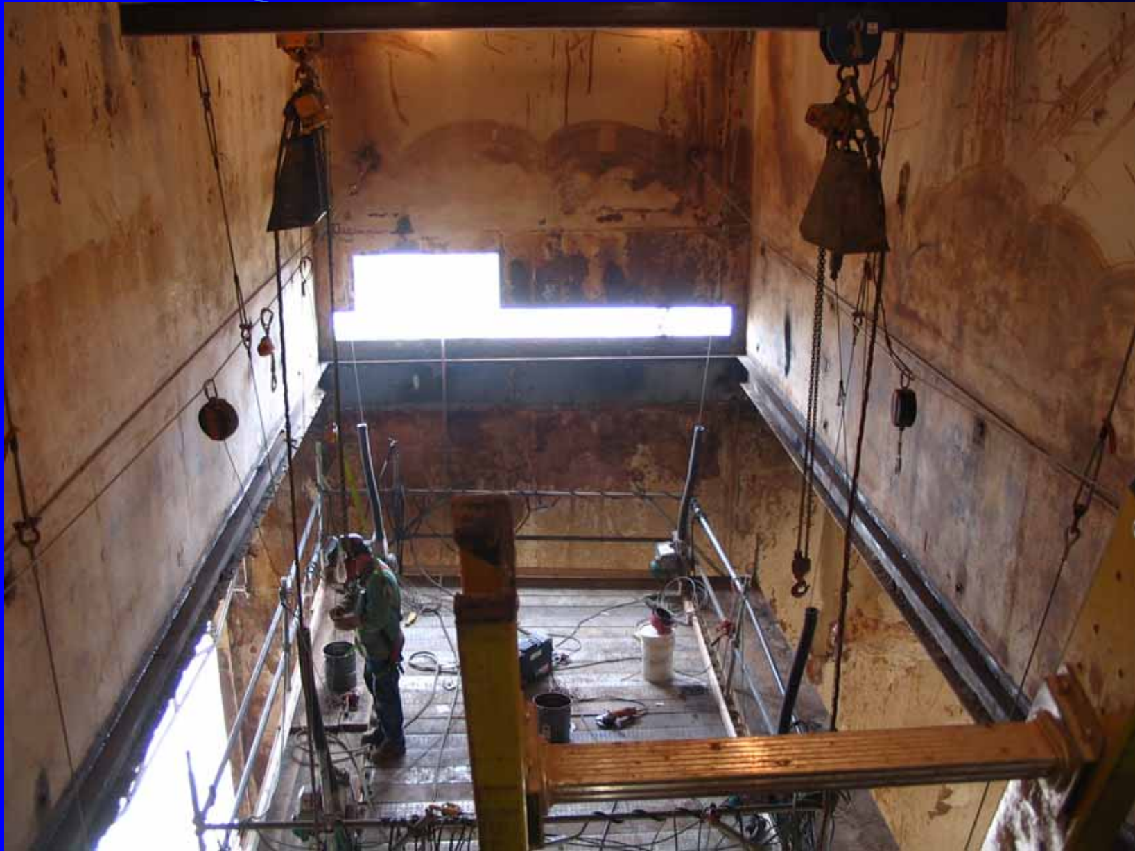
Compartment Tubesheet Shelf Installation
