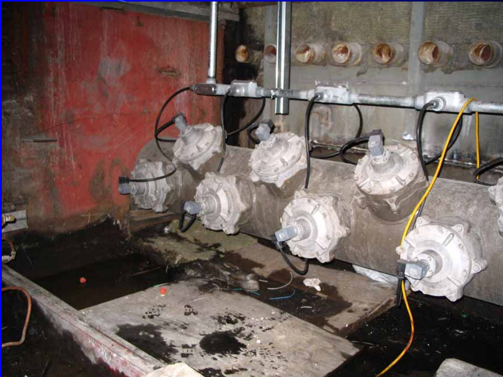
4" Pulse Valve Header Assemblies
