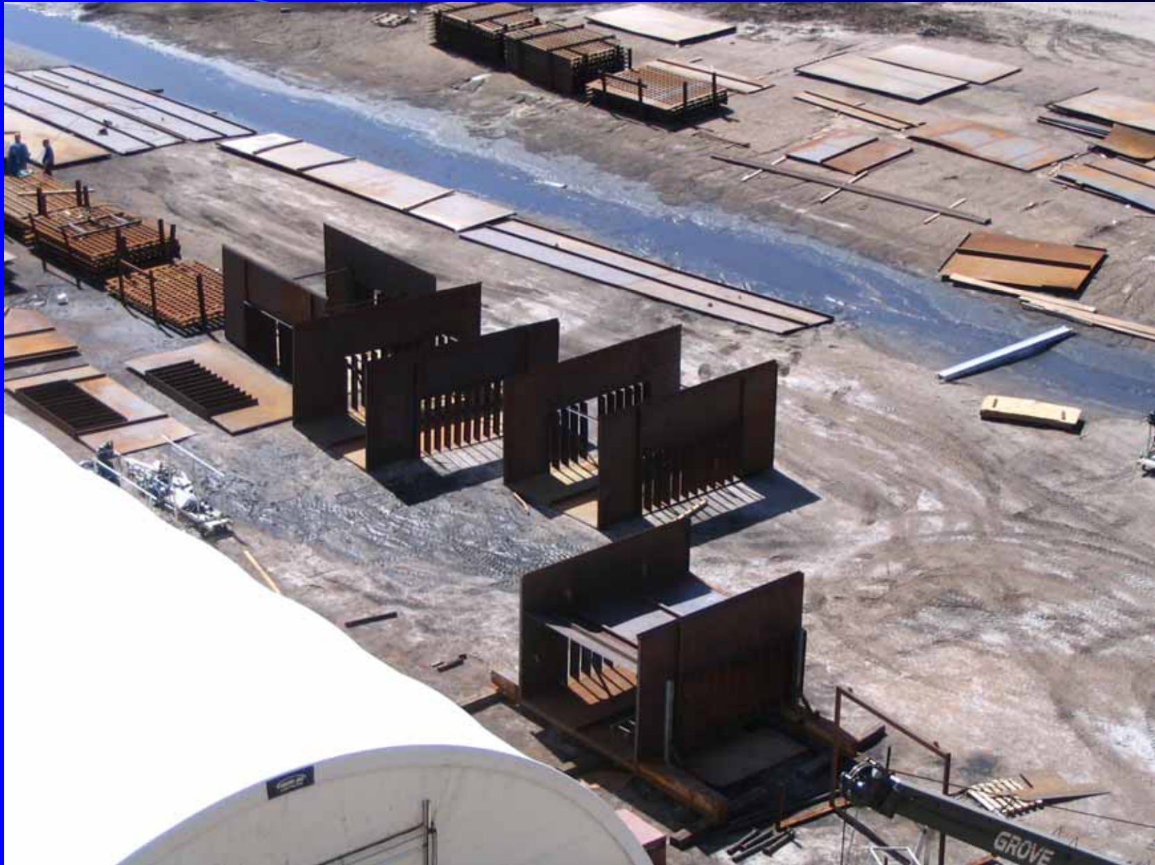
Pre-Assembly of Inlet Plenum Sections
