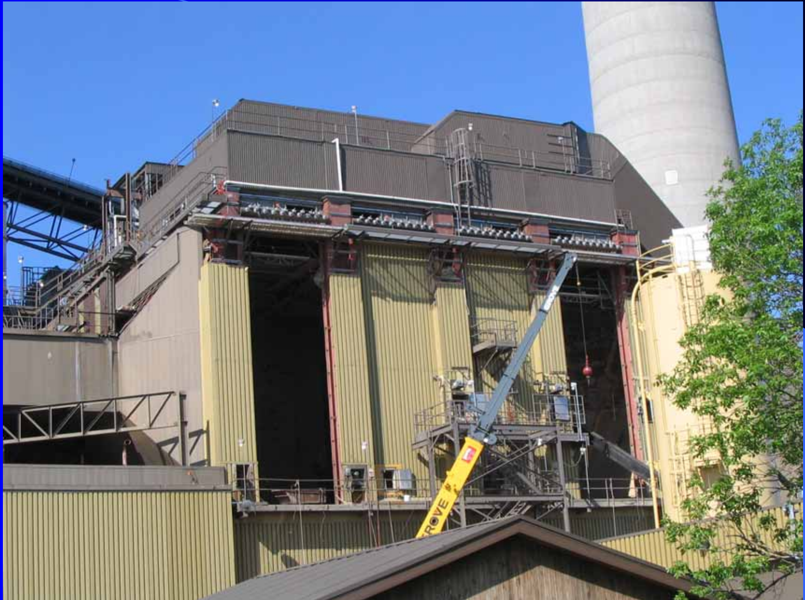
ESP Side Cut-outs for AHPC Demolition
